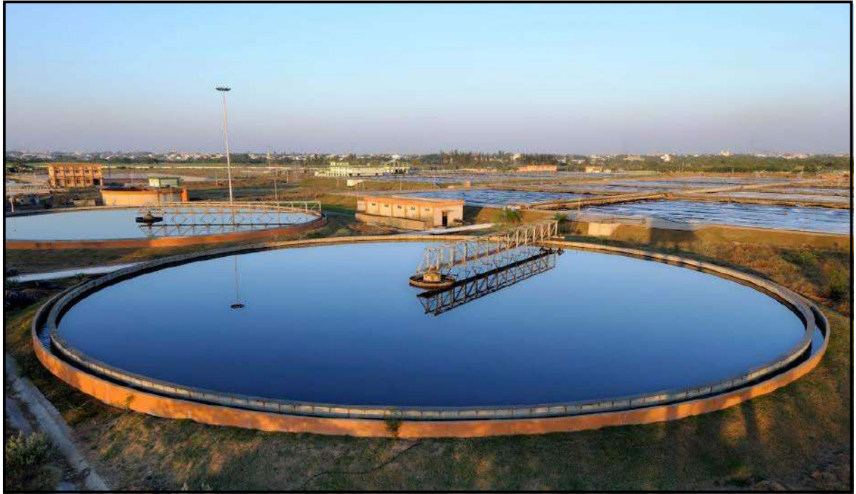
Clarifier at FETP, Ankleshwar
