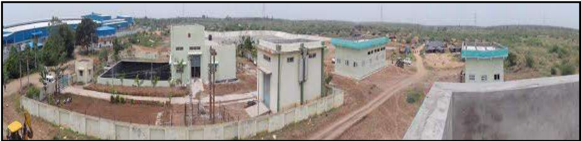
Recently Commissioned Jhagadia Pump House
